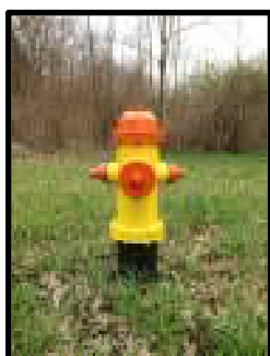
A fire hydrant painted yellow with ORANGE caps/bonnets – hydrant is capable of producing flows in excess of 500 gallons per minute.
